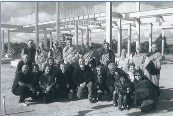
Sangha and lay community viewing progress of stage 1 steel works on International Sangha Day
